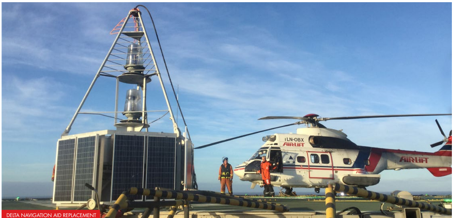
DELTA NAVIGATION AID REPLACEMENT
