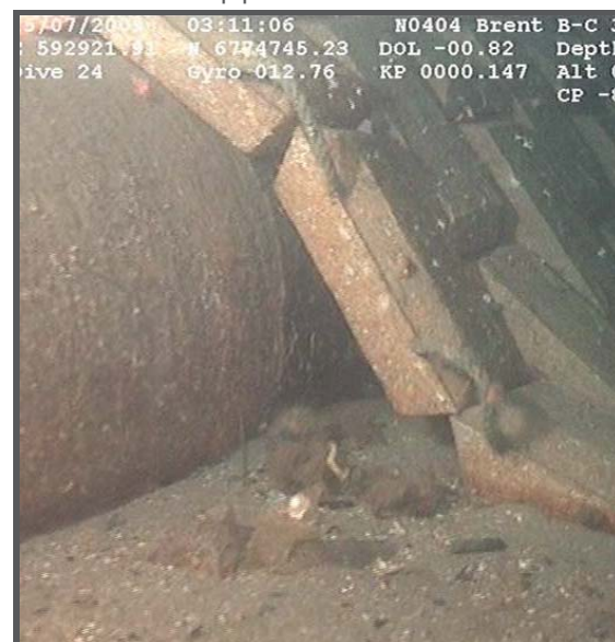
Mattress over 30" pipeline
