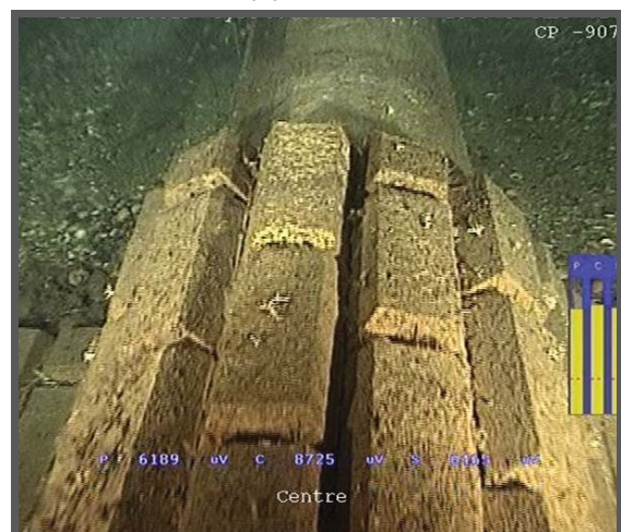
Mattresses on subsea pipeline
