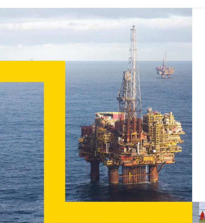
There are also considerable engineering challenges and safety risks associated with cutting through, lifting and transporting the reinforced concrete legs for removal which we are currently investigating. This type of operation – to remove gravity base structures – has never been attempted before in the North Sea.
