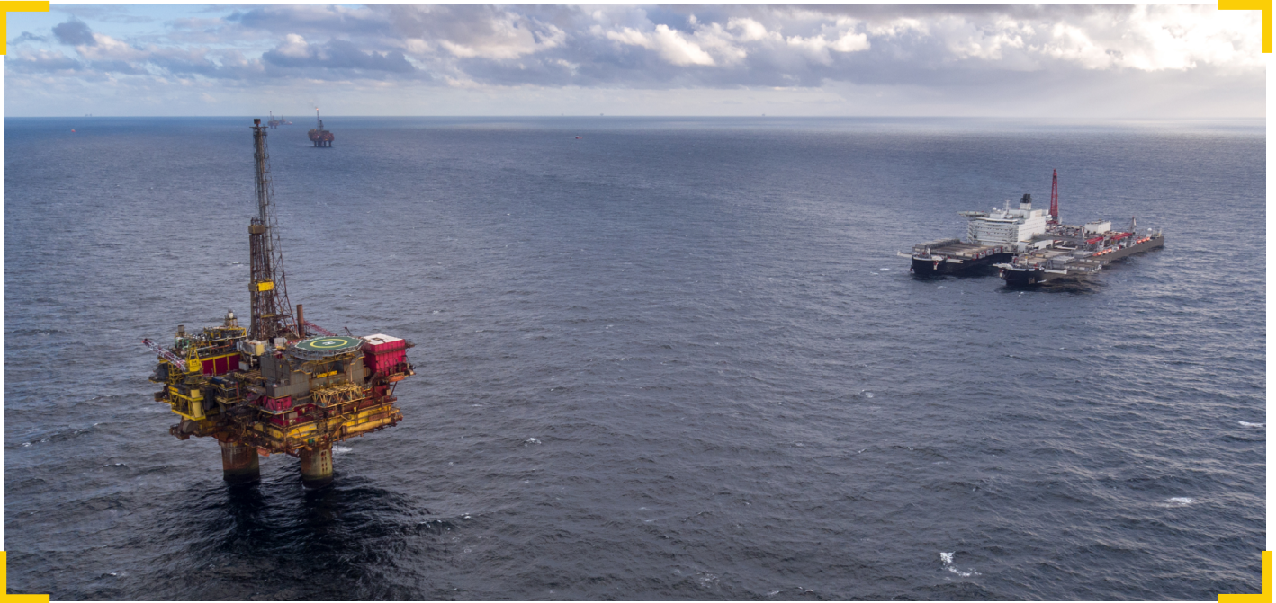
The Pioneer Spirit closes in on Brent Delta ready for the lift
