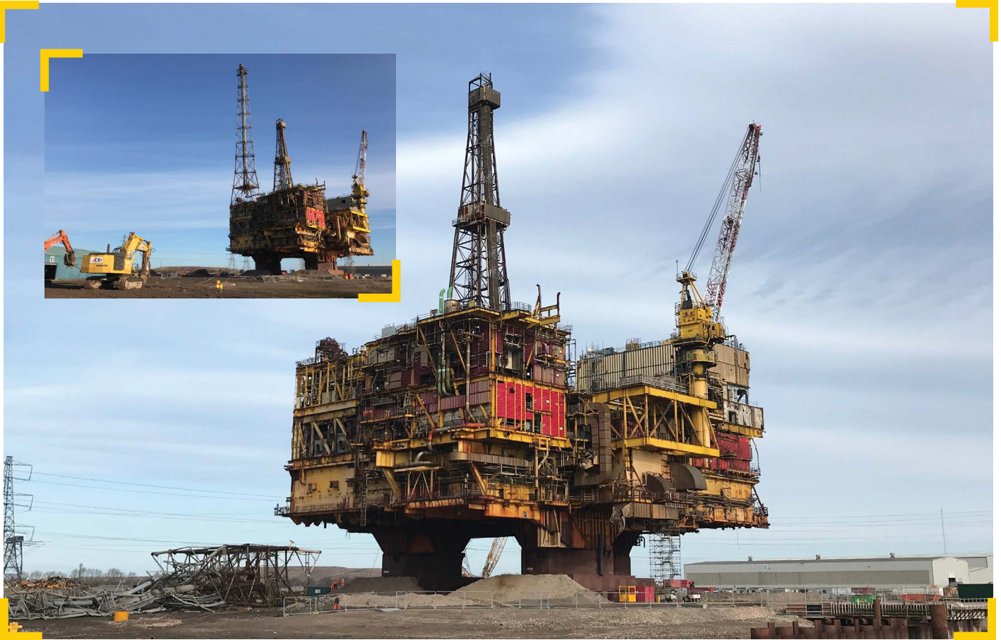
Brent Delta topside - before and after the successful removal of the flare stack at Able UK
